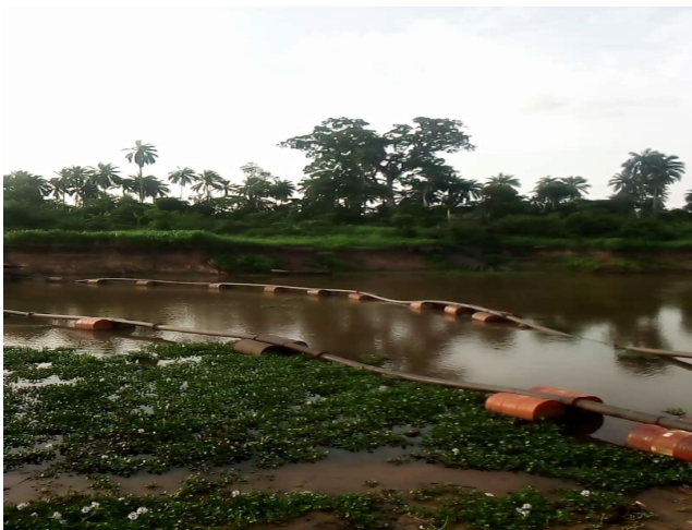
Fig 3. Uncontrolled dredging on shallow streams causing severe erosion along Igbogene-Gbrain road, Bayelsa State.
